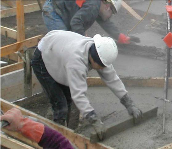
Both feet together increases reaching distance which is hard on the back and shoulders.
