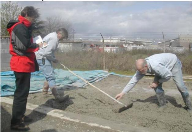
**With a 1" slump, pull forces averaged 46 pounds** with the greatest force being 60 pounds and the least being 36. These forces through the course of a day can be hard on the back and shoulders.
